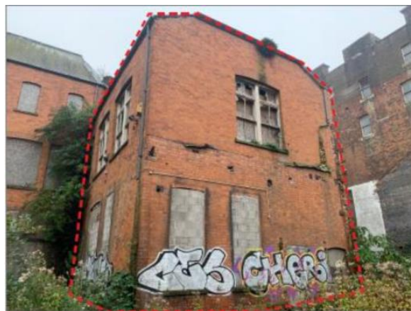
--- Areas of demolition
